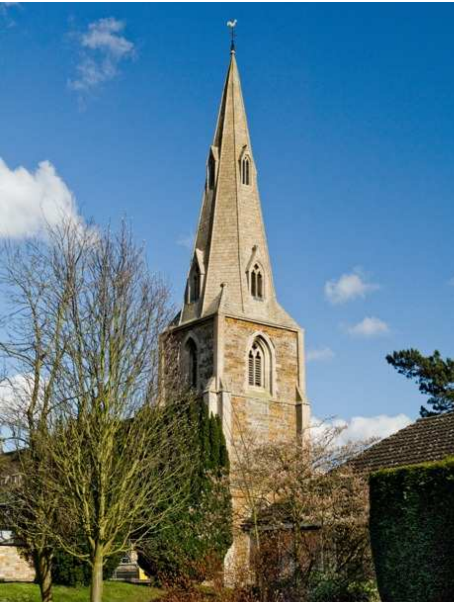
St. Peter's Church, High Street (Grade I listed)
