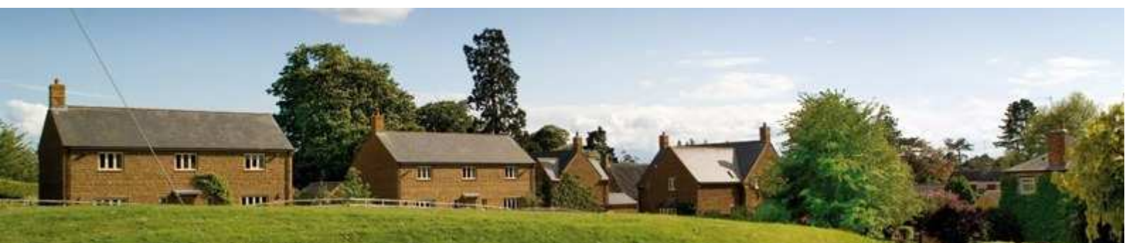
Slate roofs, looking over Paddock Close
